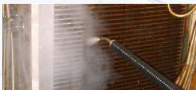
Cleaning heat exchanger.
